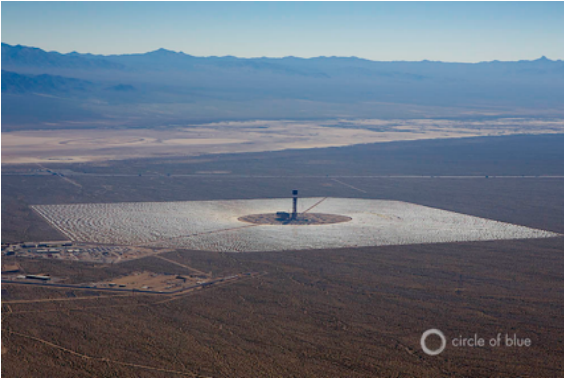
Ivanpah Solar Electric Generating System, California. Photo © J. Carl Ganter / Circle of Blue
