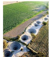
The Cantalloc Aqueducts, built by the Nazca people in the Peruvian desert 1,500 years ago, are still in use today. The uniquely shaped holes allow wind to blow into a series of underground canals, forcing water from underground aquifers into areas where it is most needed. More images/info: <a href="https://cutt.ly/aJCbVAp">https://cutt.ly/aJCbVAp</a>
