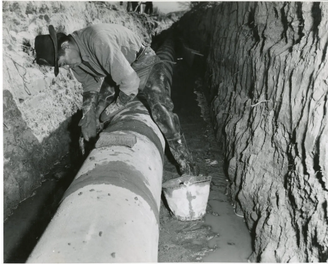
Original Caption: “Santa Clara Indian Reservation, Santa Fe, New Mexico. December 2, 1940. A member of the CCC ID crew cementing the joints in a pipe line which is being built on the Santa Clara Pueblo lands for the purpose of diverting irrigation and drinking water to the pueblo lands and surrounding areas.” Photo by WJ Mead. Local Photo ID: 35-G-17C-2077
